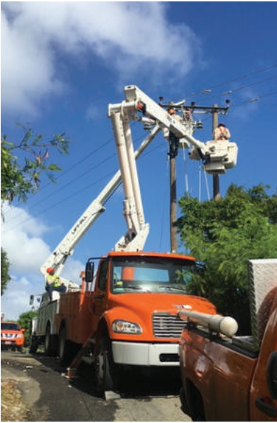
Figure 1: Work being carried out in Hannah's Estate December 2016 by Distribution Linesmen
